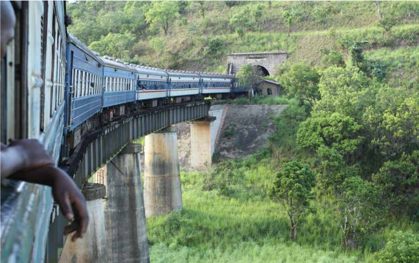
Tazara railway line
